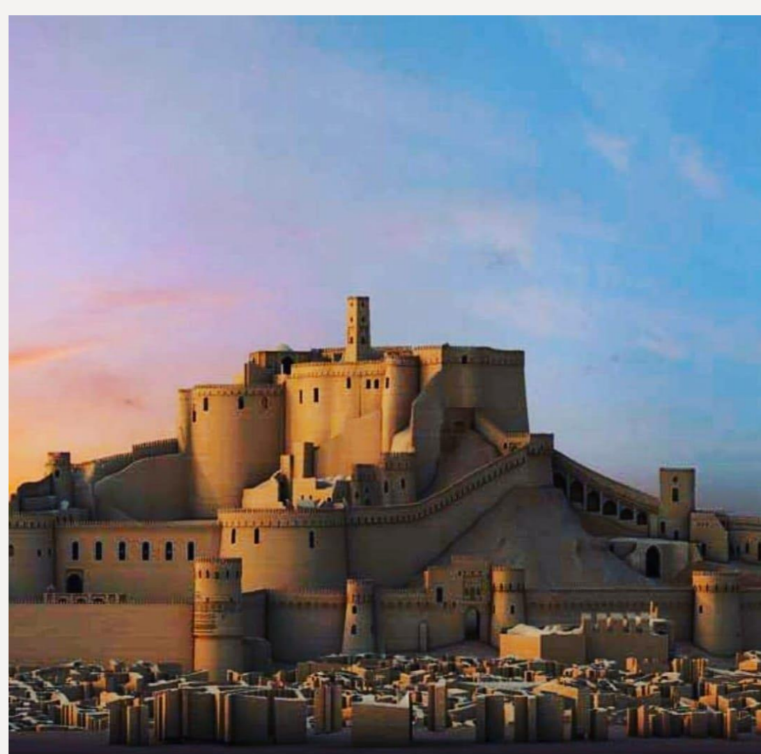
Fig 1. Arg-e Bam, the largest adobe building in the world. Bam, Kerman, Iran
