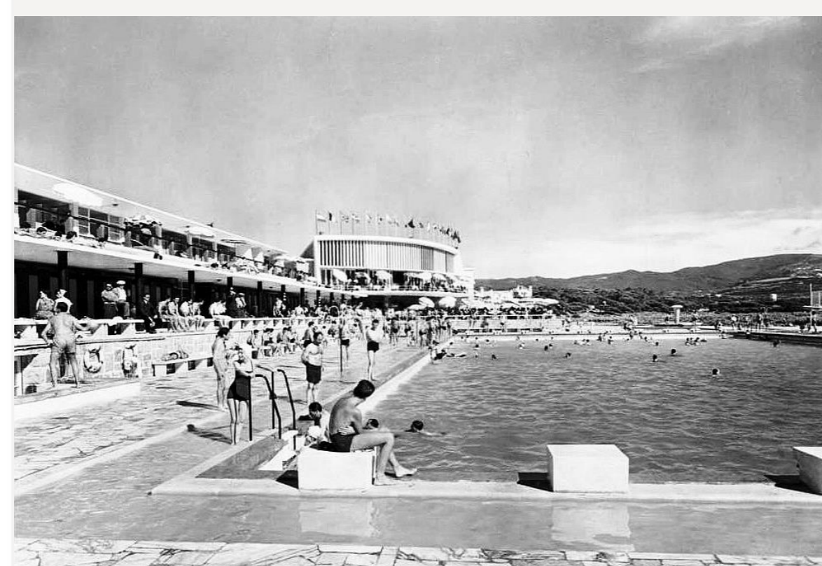
Swimming pool and restaurante Concha, Praia das Maças, 1955. Arquivo Municipal de Lisboa
