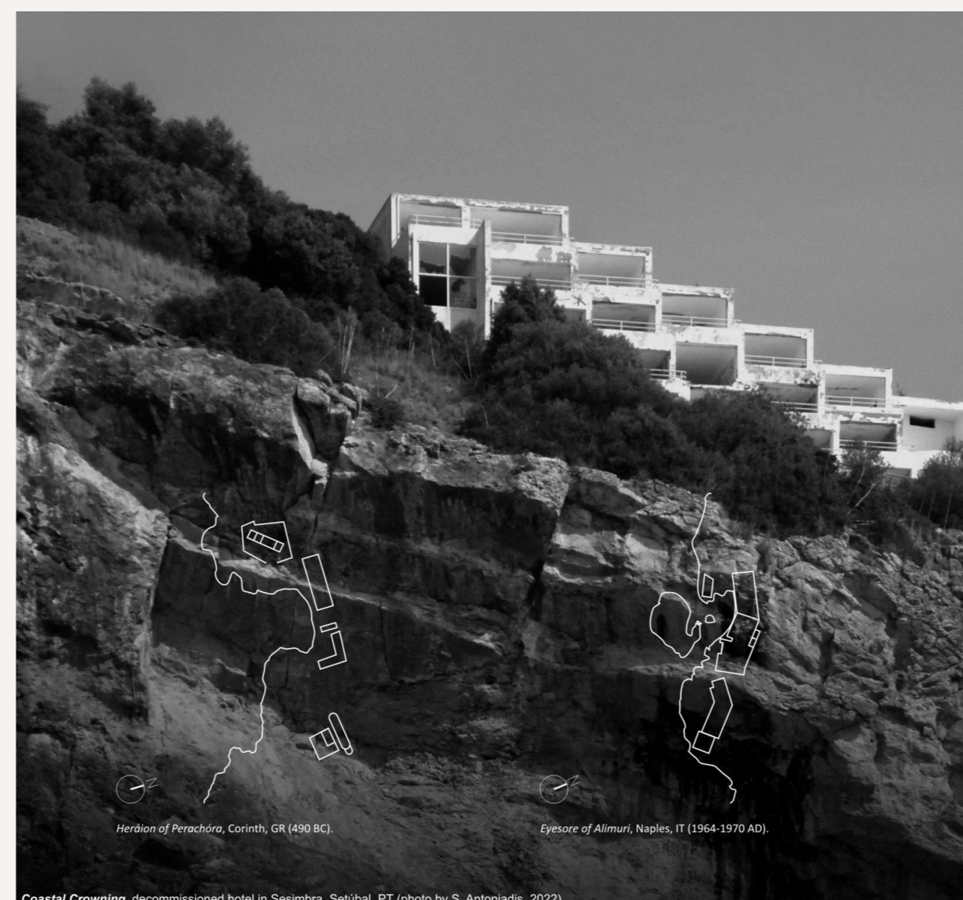
Coastal Crowning, decommissioned hotel in Sesimbra, Setúbal, PT (photo by S. Antoniadis, 2022).
